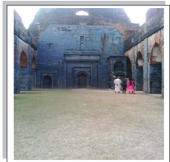
Fig - Central Nave, Adina Mosque
